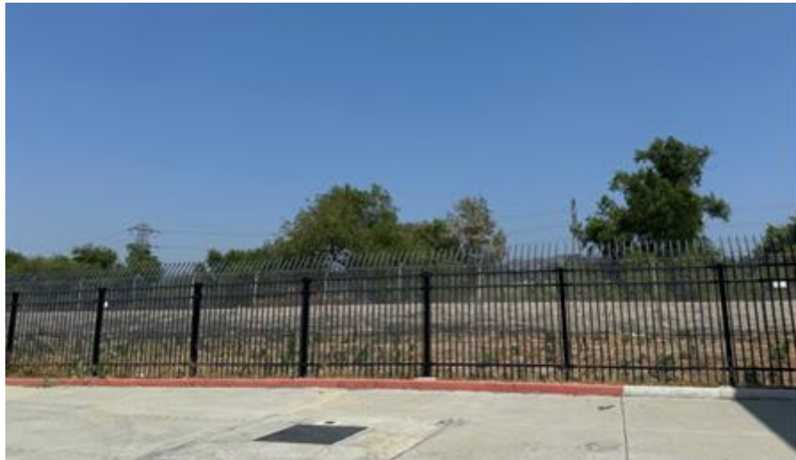
Figure 9-5: ARC Perimeter Berm
