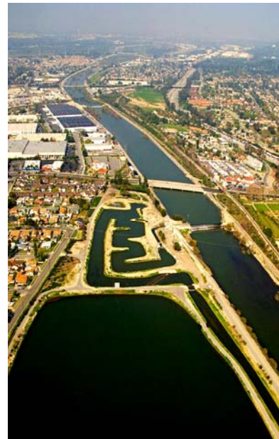
A wet period along the San Gabriel River groundwater replenishment area
