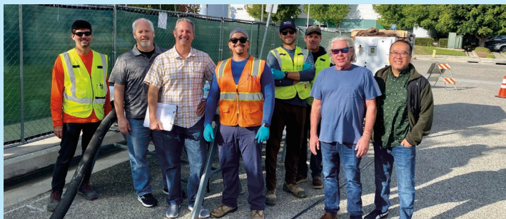
Aquifer testing is underway in the South Bay as part of WRD's Brackish Groundwater Reclamation Program.
