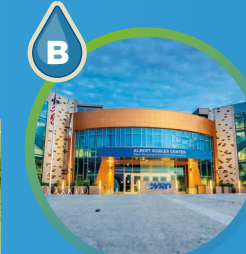
Albert Robles Center for Water Recycling & Environmental Learning (ARC)
