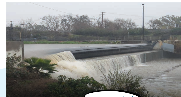
The San Gabriel River Rubber Dam is part of the infrastructure that helps us capture stormwater while maintaining flood control functions. The picture is from the February 5, 2024 storm.
