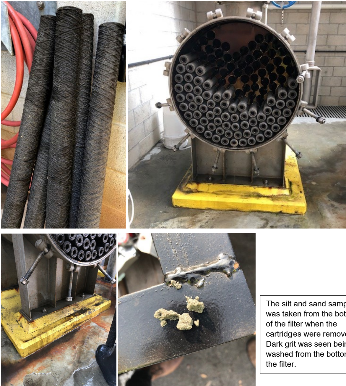
Figure 2-9. Cartridge Filters during Replacement on September 16, 2020
