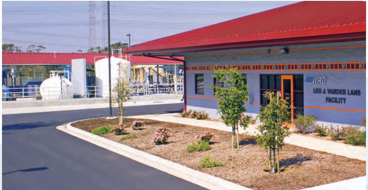
WRD's Leo J. Vander Lans Advanced Water Treatment Facility in the City of Long Beach
