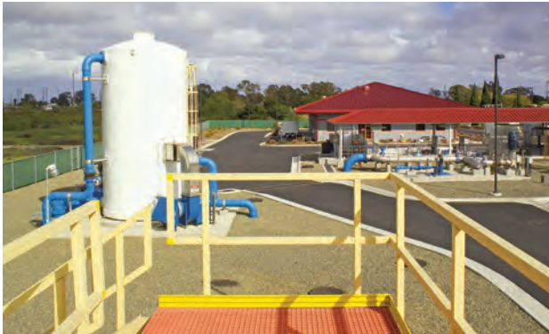
Leo J. Vander Lans Advanced Water Treatment Facility
