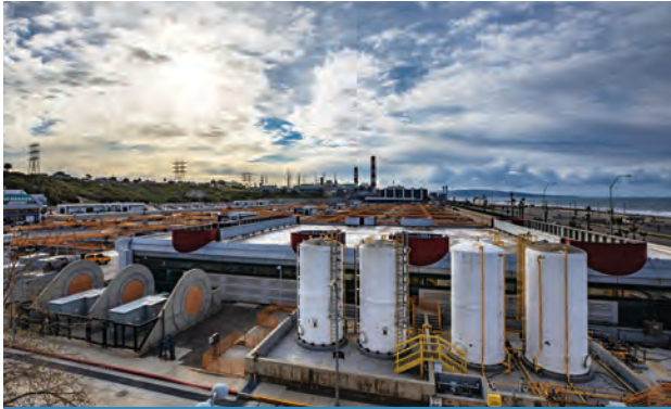
Hyperion Water Reclamation Plant Image courtesy of the City of Los Angeles
