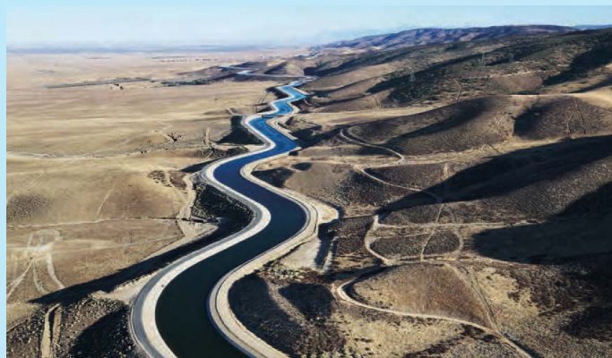
Photo of California's aqueduct. The aqueduct is a series of canals, pipelines and tunnels that bring water hundreds of miles to LA County.
