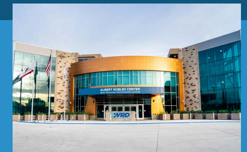
2019 - WRD celebrates the grand opening of the Albert Robles Center, a water purification plant that treats up to 14.8 million gallons of water per day.
