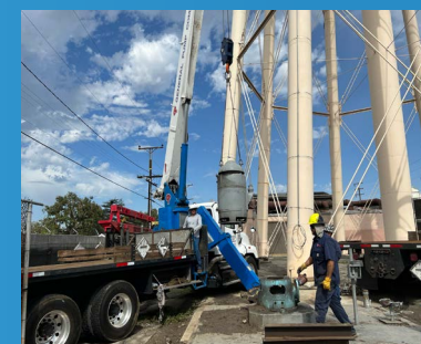
WRD working to destroy an inactive water supply well.
