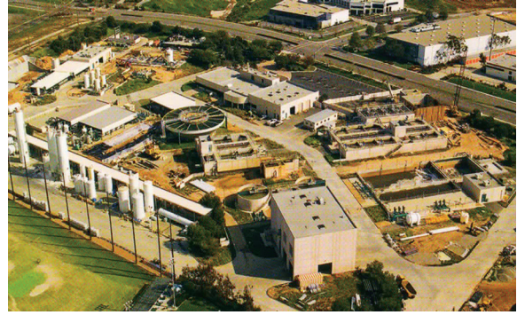
West Basin Municipal Water District's Edward C. Little Water Recycling Facility in El Segundo, CA, 1995. Image courtesy of West Basin Municipal Water District.
