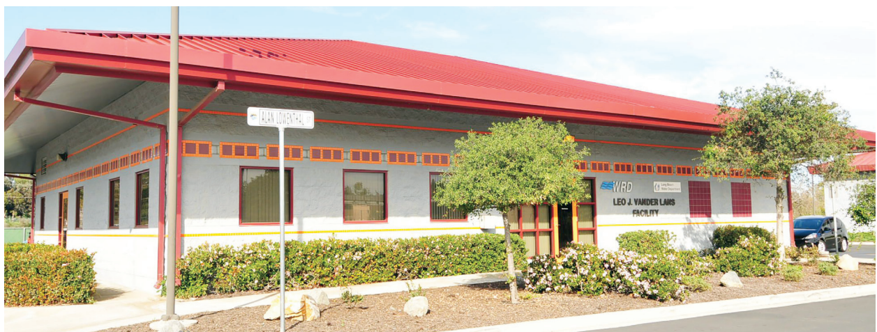
WRD's Leo J. Vander Lans Advanced Water Treatment Facility in the city of Long Beach, 2015. Image from the WRD archives.
