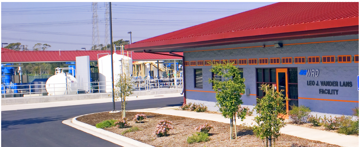
WRD's Leo J. Vander Lans Advanced Water Treatment Facility, Long Beach, 2015. Image from the WRD archives.
