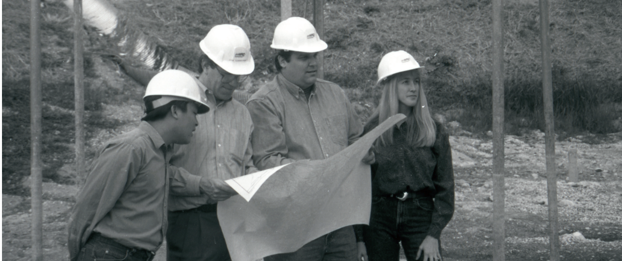
Robb Whitaker with WRD Engineers Mario Garcia, Jim Leserman and Melinda Sperry view construction at the Leo J. Vander Lans Advanced Water Treatment Facility, 2001. Image from the WRD archives.
