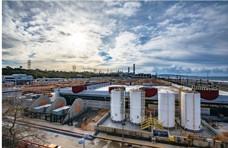
Hyperion Water Reclamation Plant, Los Angeles, ca. 2000. Image courtesy of the city of Los Angeles.
