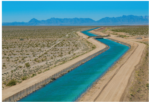
Colorado River Aqueduct, transporting water through the Mojave Desert, ca. 1970s. Image courtesy of Metropolitan Water District of Southern California.
