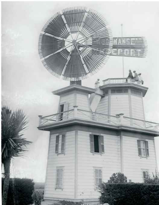
A windmill used to pump water for irrigation, Compton California, ca 1900. Image courtesy of USC Digital Library - California Historical Society Collection.
