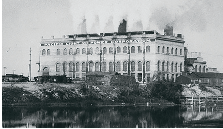
The Pacific Light and Power Co. Steam Plant in Redondo Beach, 1912. In 1917, Pacific Light and Power Co. was acquired by Southern California Edison. Image courtesy of Daily Breeze.
