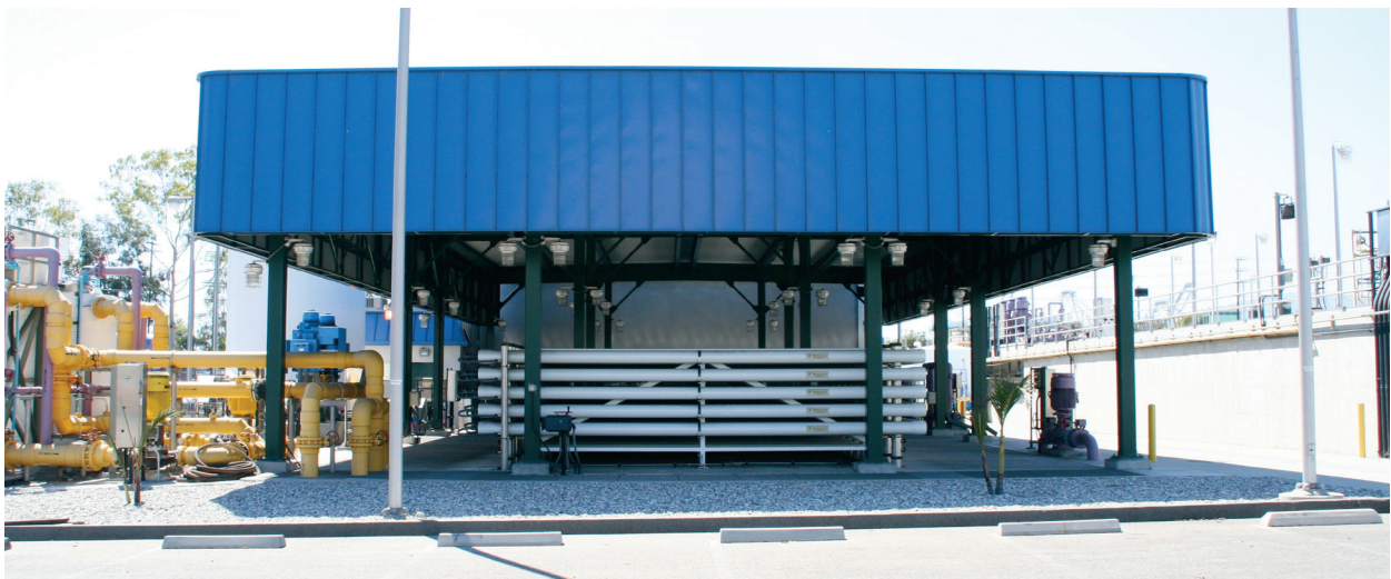
City of Los Angeles Terminal Island Advanced Water Purification Plant, completed in 2006 to provide recycled water to the Dominguez Gap Barrier. Image courtesy of the City of Los Angeles.
