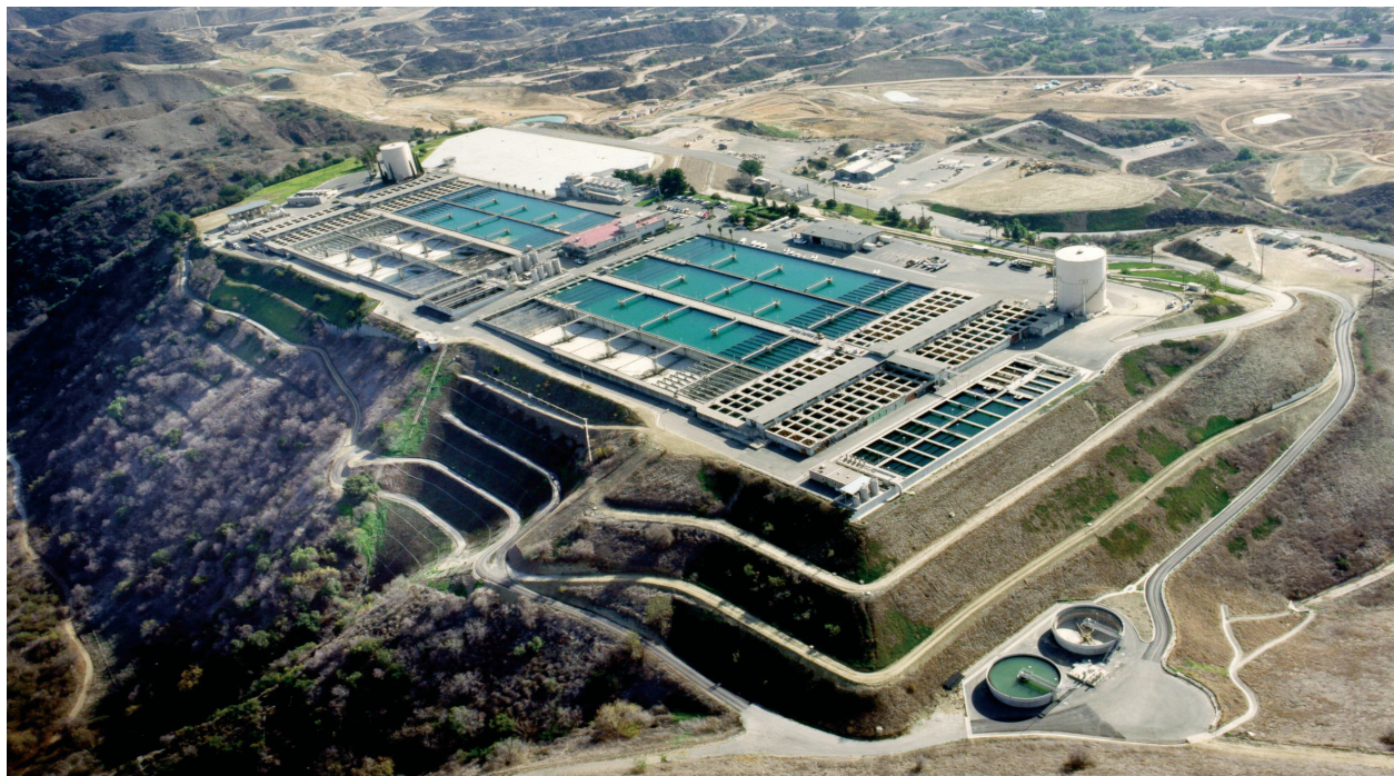
Metropolitan Water District's Diemer Treatment Plant in Orange County, 1963. Image courtesy of Metropolitan Water District of Southern California.
