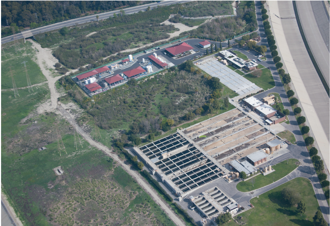
Aerial view of the Los Angeles County Sanitation Districts' Long Beach Water Reclamation Plant (foreground) and WRD's Leo J. Vander Lans Advanced Water Treatment Facility (red-roofed structures), 2015. Local wastewater is treated at the water reclamation plant before further treatment at the advanced water treatment facility. Image from the WRD archives.
