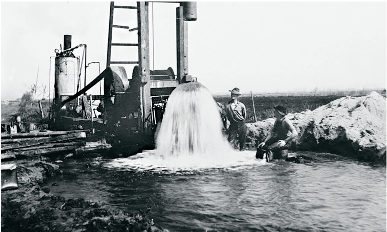
Artesian well in northern Long Beach early in the twentieth century. The aquifer that runs parallel to the San Gabriel and Los Angeles Rivers once produced more than a thousand artesian wells that flowed like this one. Image courtesy of the Security Pacific National Bank Collection – Los Angeles Public Library.
