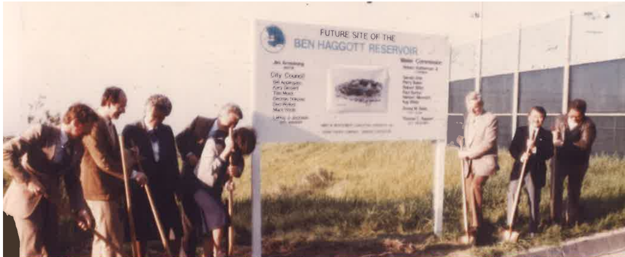
Haggott Reservoir in Torrance approximately half complete at a groundbreaking event, ca. 1986. Image courtesy of the city of Torrance.
