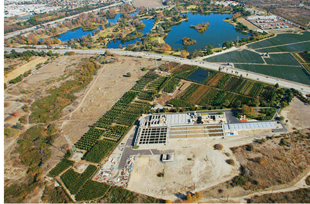
Whittier Narrows Water Reclamation Plant, 2006. Image from the WRD archives.
