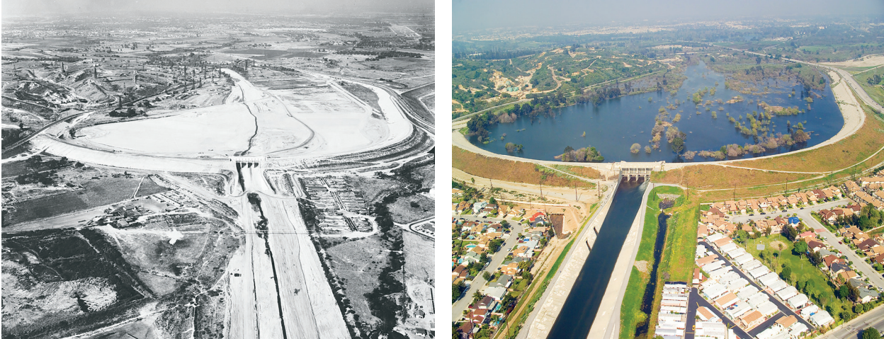
Whittier Narrows Dam Project while under construction, ca. 1957 (left) and filled with captured stormwater in 2007 (right). Images from the WRD archives.
