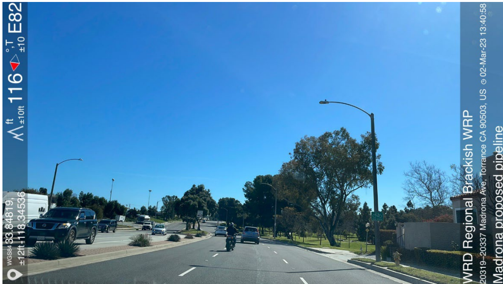
Photo 10 (S). Representative photograph of the Proposed Brine Disposal Pipeline, along Madrona Avenue.
