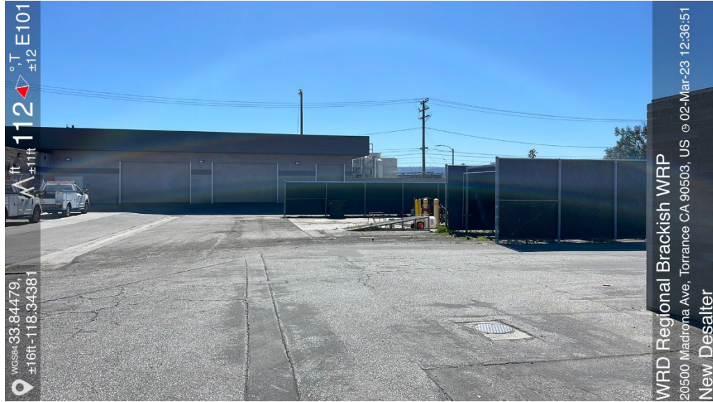
Photo 15 (S). Representative photograph of the Treatment Facility Site.
