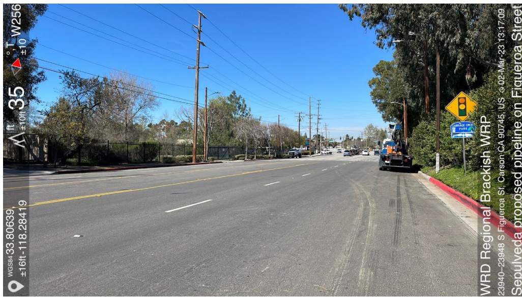
Photo 12 (N). Representative photograph of the Proposed Brine Disposal Pipeline, along Figueroa Street.
