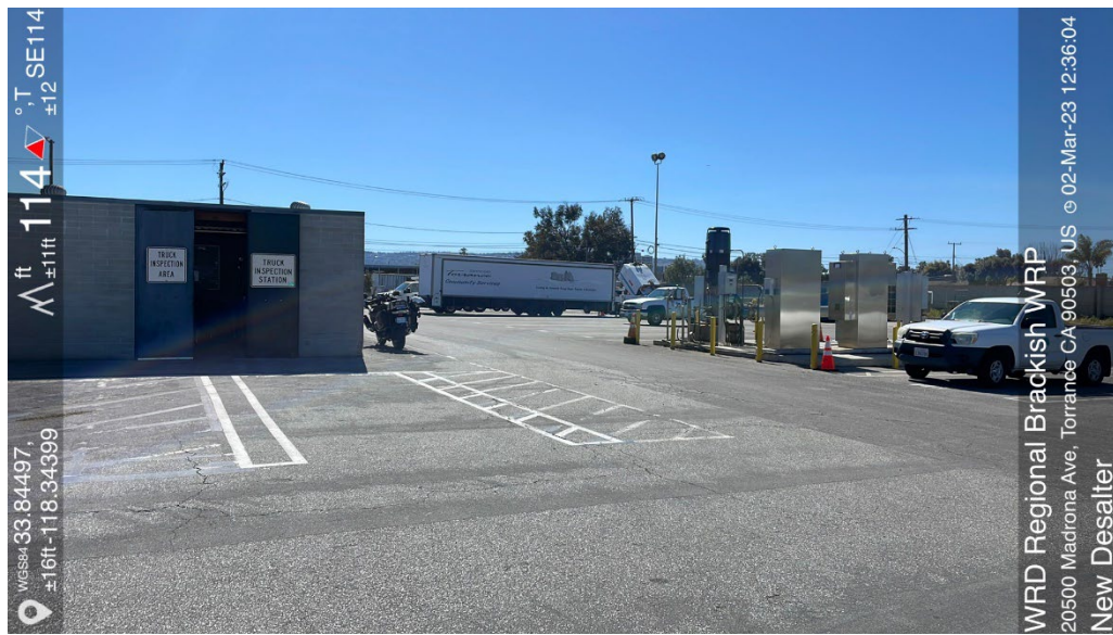
Photo 16 (SE). Representative photograph of the Treatment Facility Site.
