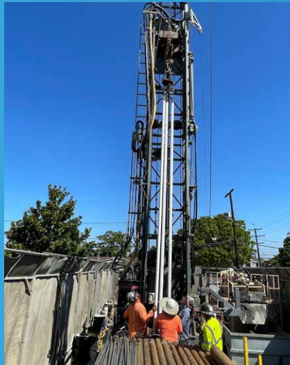
This monitoring well, located at La Romeria Park in Torrance helps WRD's hydrogeologist track the levels of groundwater in aquifers.
